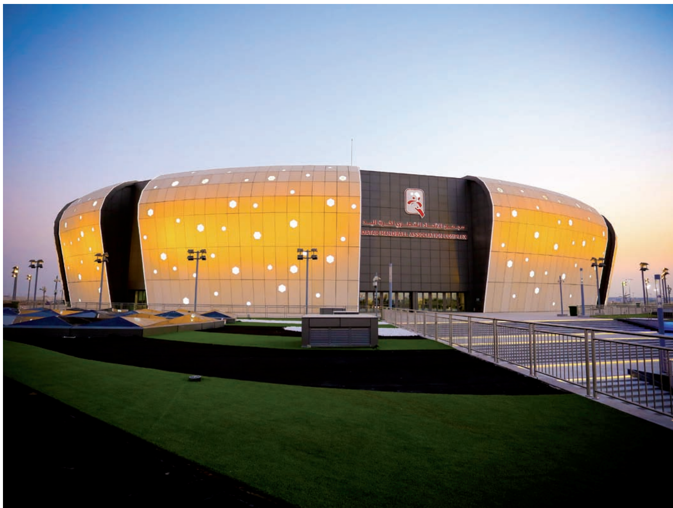
Qatar Handball Association Complex, Doha, Qatar
